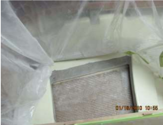
Starboard pan liner cut out, below chain plate,
