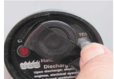
Fire extinguisher control with unresponsive indicator
