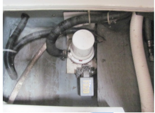
Accommodation space bilge
