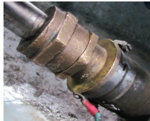
Starboard stuffing box
